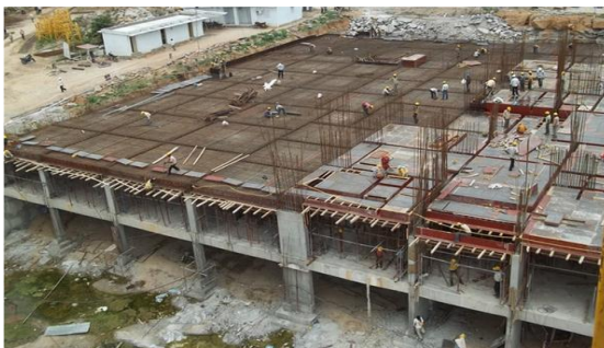
Fig. No.1 Conventional Formwork.
